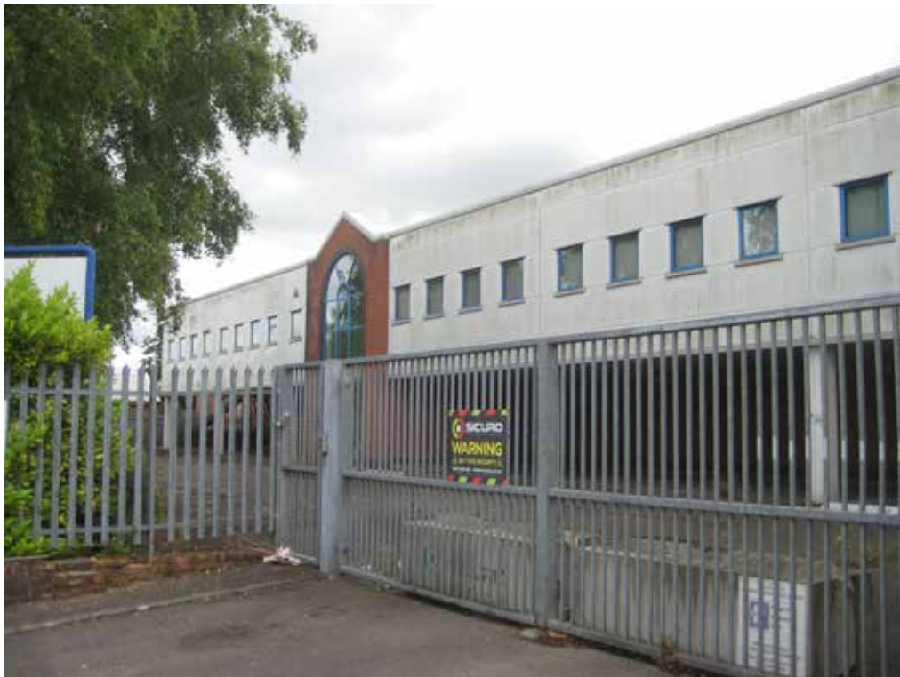
Unit 6 viewed from Rowanfield Road
