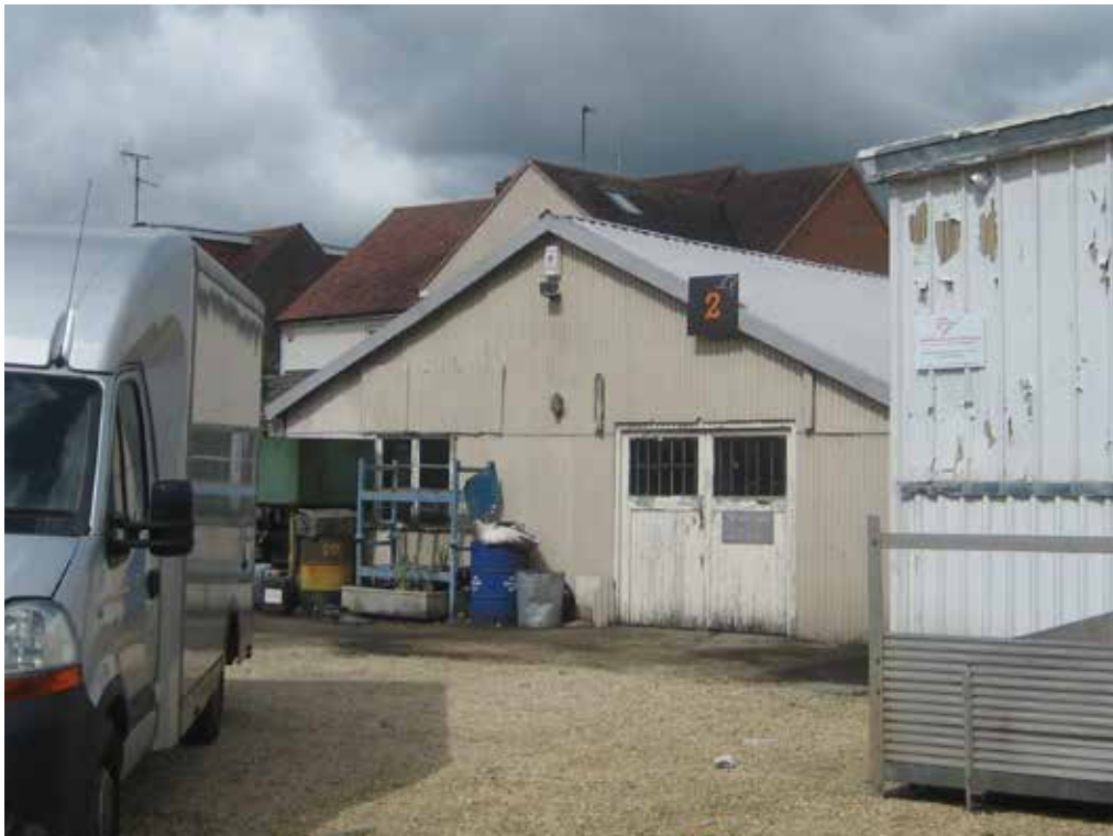
Unit 2 viewed from the south east
