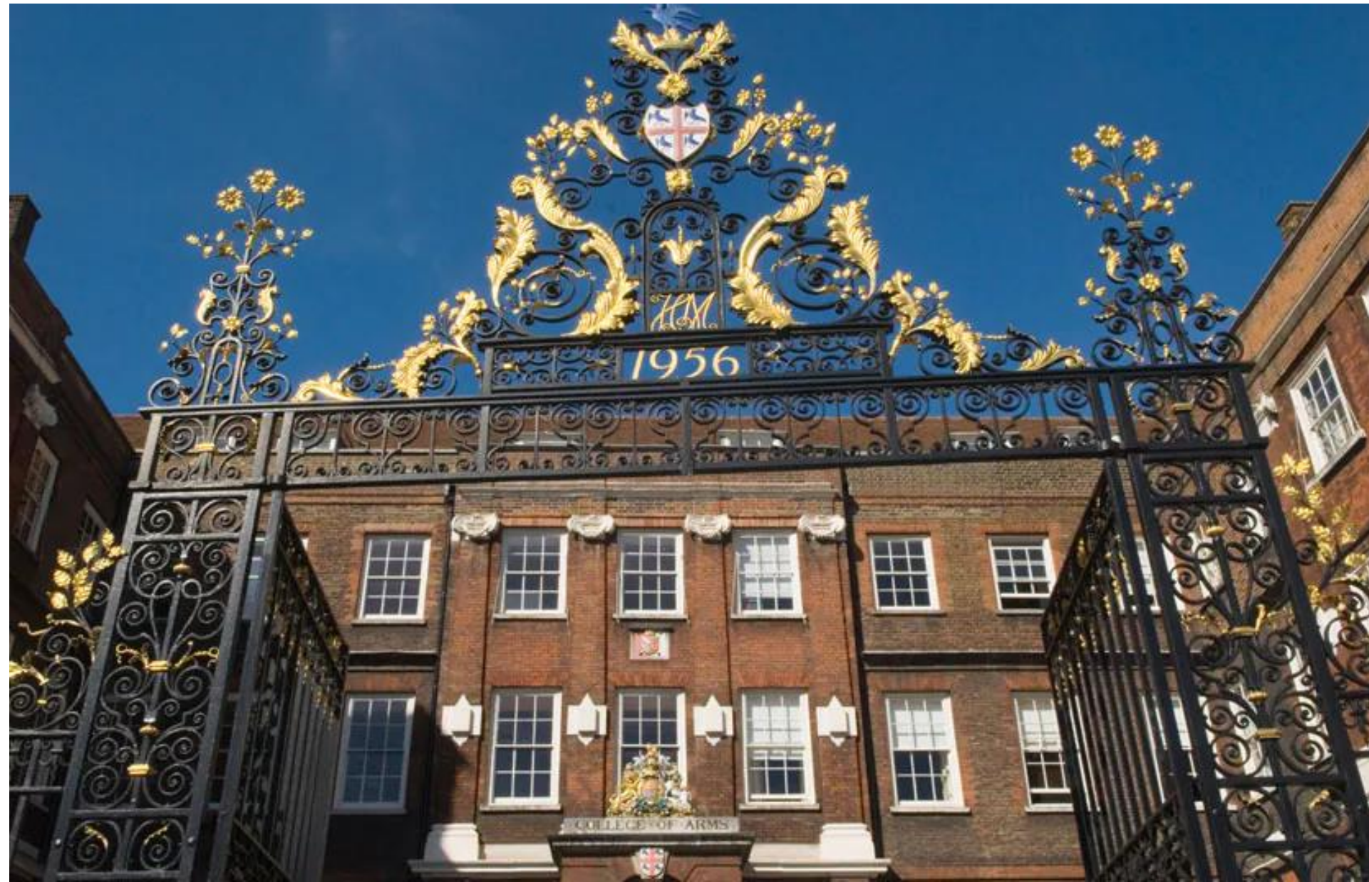
College of Arms Railings and Gates, London. Originally at Goodrich Court (Grade I)
