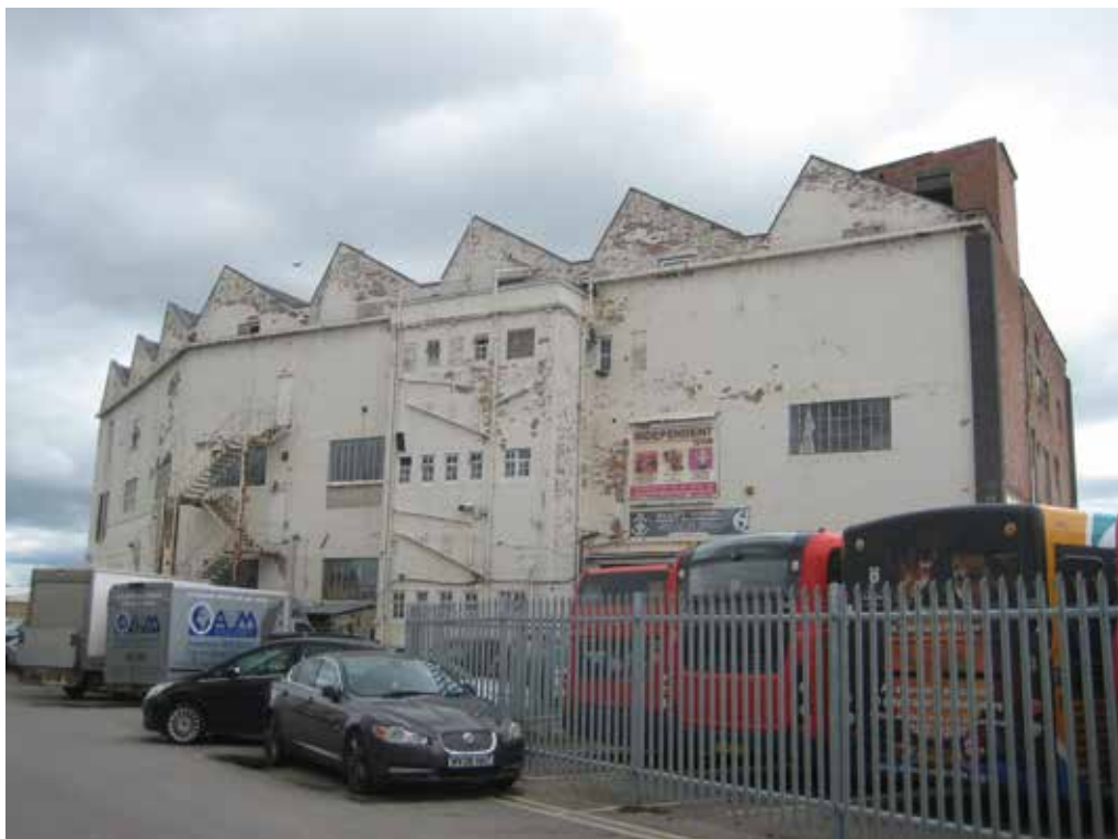
Unit 2 viewed from Rowanfield Road
