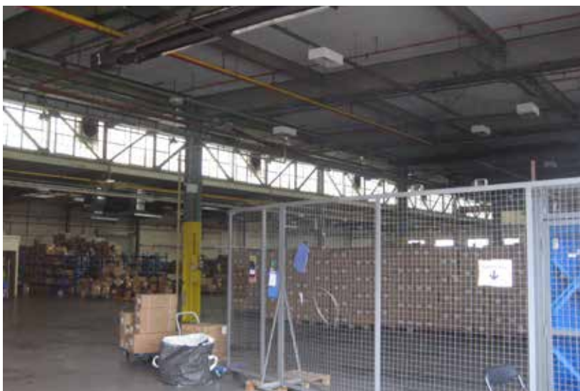
Internal view of Unit 8
