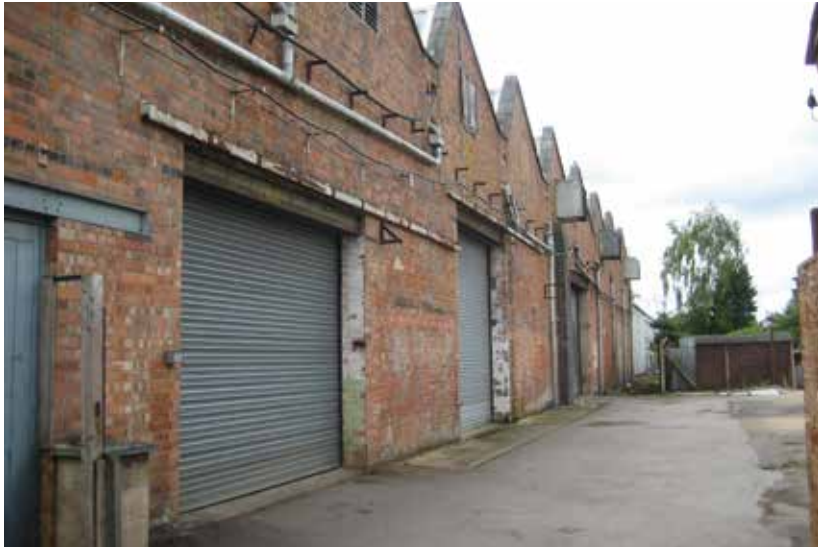
View south-westwards along the north-western elevation of Unit 1
