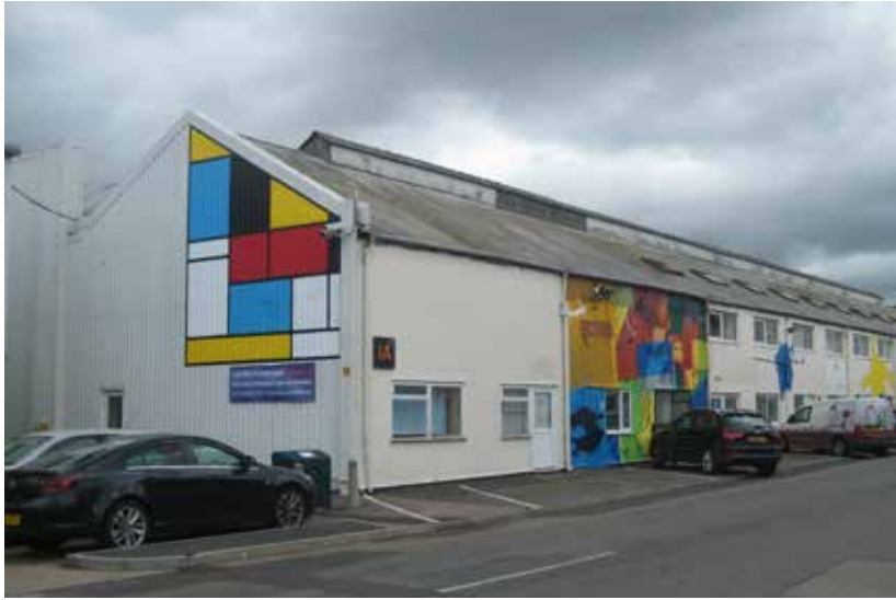
View of the pitched-roofed range (Unit 1A) abutting the south-eastern side of the northlight building (Unit 1)
