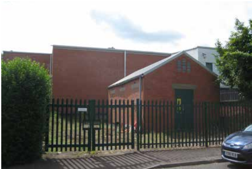
The northern end of Unit 6 viewed from Rowanfield Road; the building in the foreground is an electrical substation
