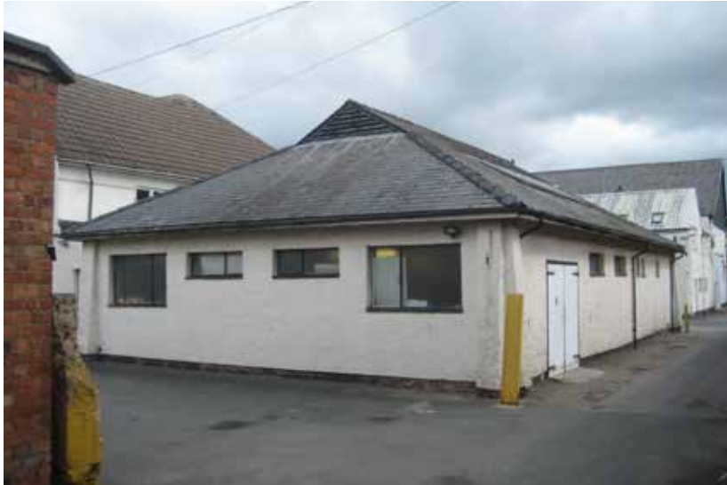
Unit 4 viewed from the south west
