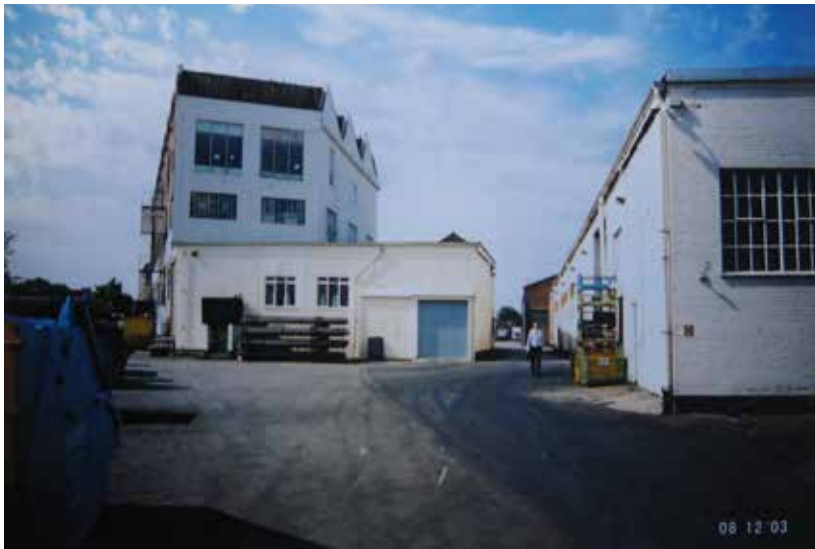
The single-storey extension at the northern end of Unit 11, photographed in 2003
