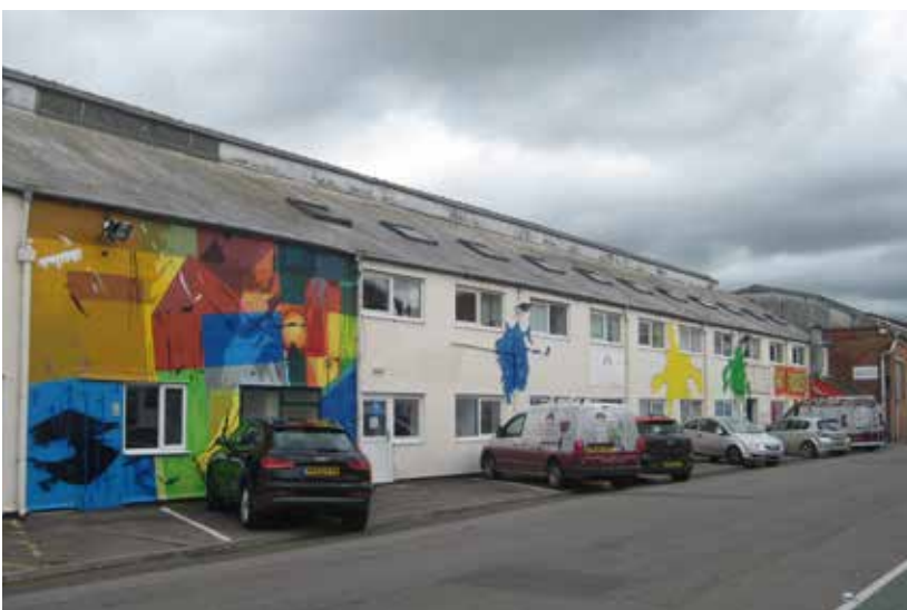
The south-western side of Unit A1 looking north; the present fenestration is modern
