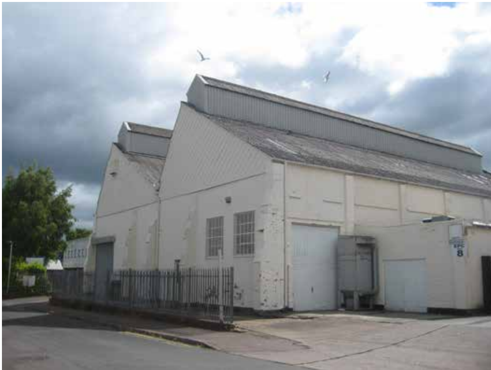
Unit 5 viewed from Rowanfield Road
