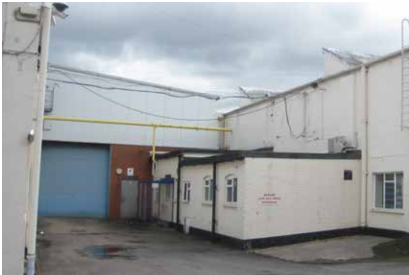
Unit 6 viewed from the southwest between Unit 5 (left) and Unit 8 (right)
