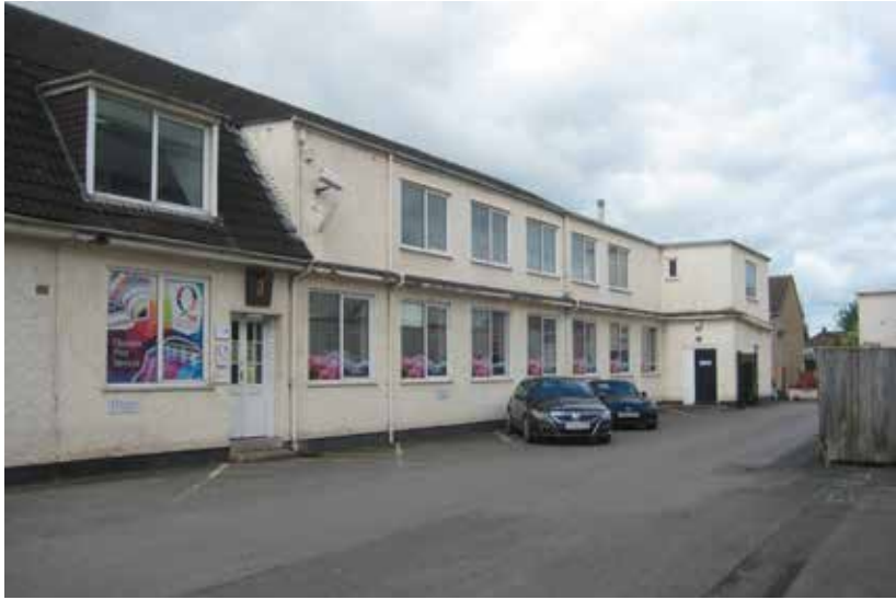
Unit 3 viewed from the south east
