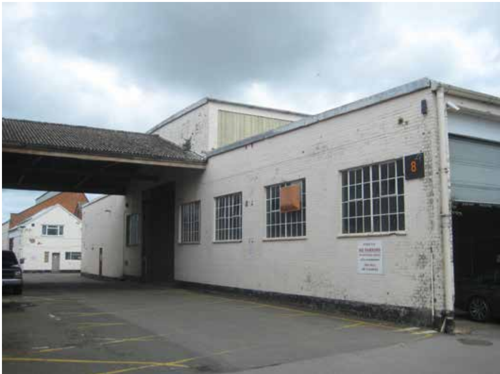
Unit 8 viewed from the south
