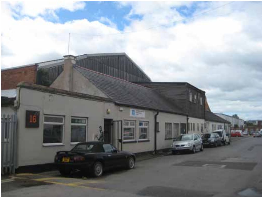
Units 15-17 viewed from the north east
