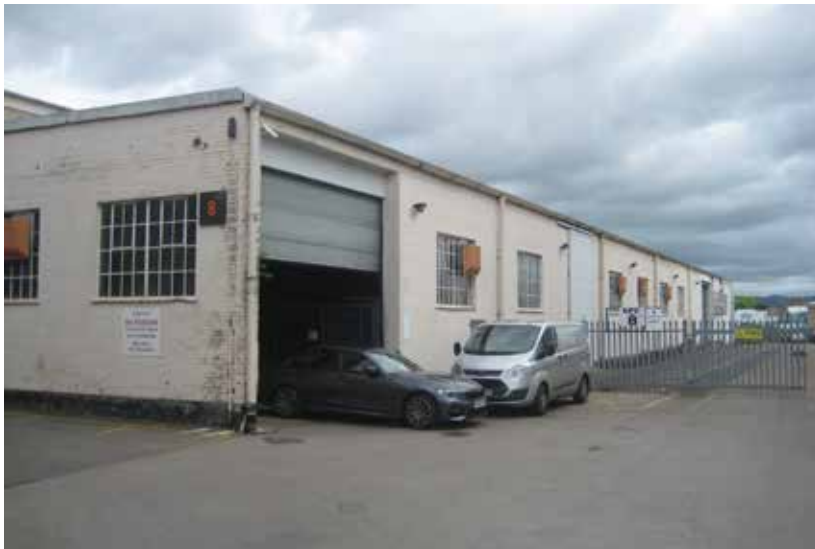
The south-eastern elevation of Unit 8
