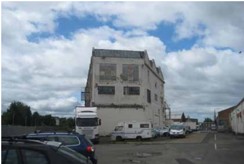
The northern end of Unit 11
