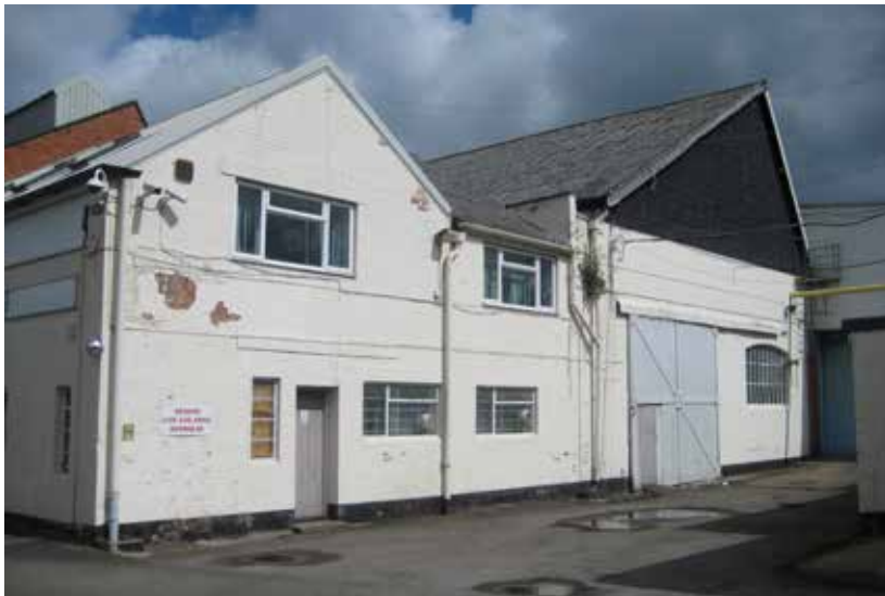
The remodelled south-eastern end of Unit 5
