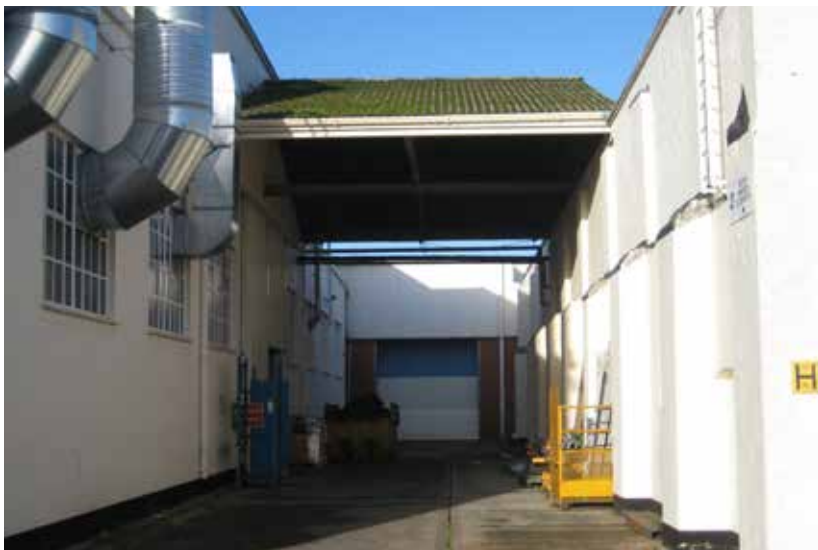
View of the covered way between Unit 8 (left) and Unit 7 (right) towards the rear of Unit 6
