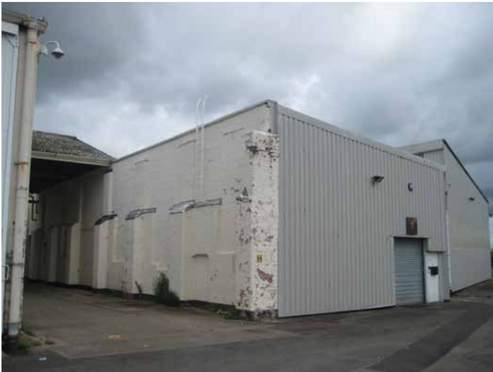
Unit 7 viewed from the south
