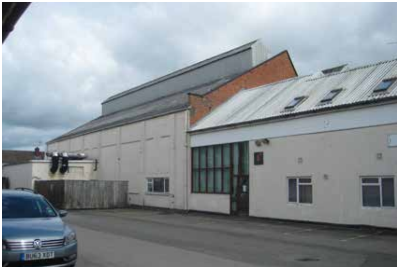
View of the south-western side of Unit 5
